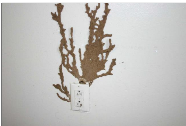
Subterranean termite shelter tubes.
